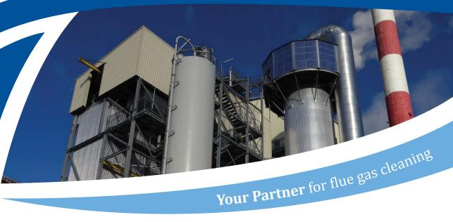
SEMI-DRY FGD : **Conditioned SecoLAB**® process operated with quick or hydrated lime for high reliability and availability
